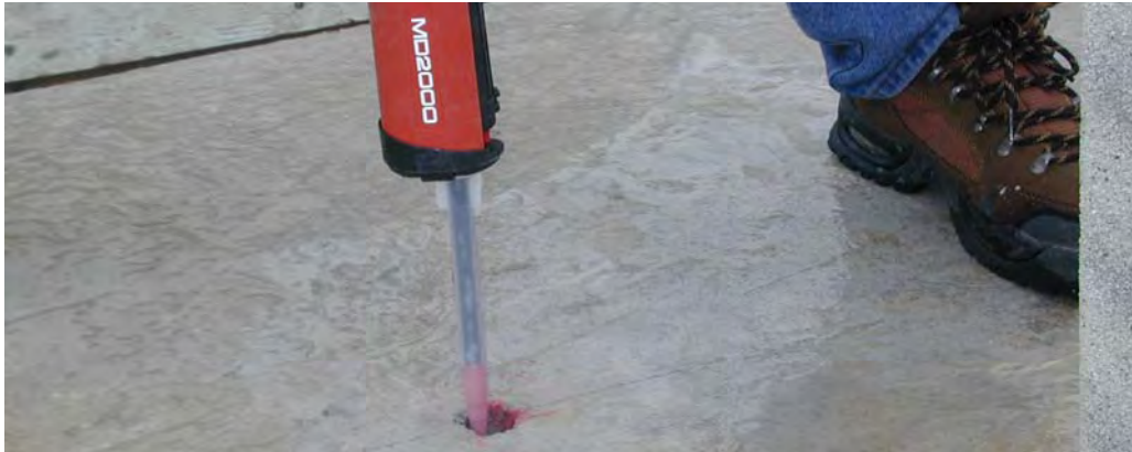
Figure 4: Injection of the Adhesive into the Hole
