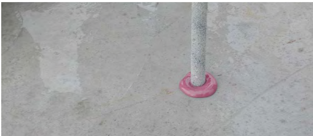
Figure 5: Installing the Bar
