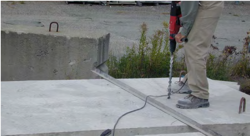
Figure 2: The Drilling of the Holes
