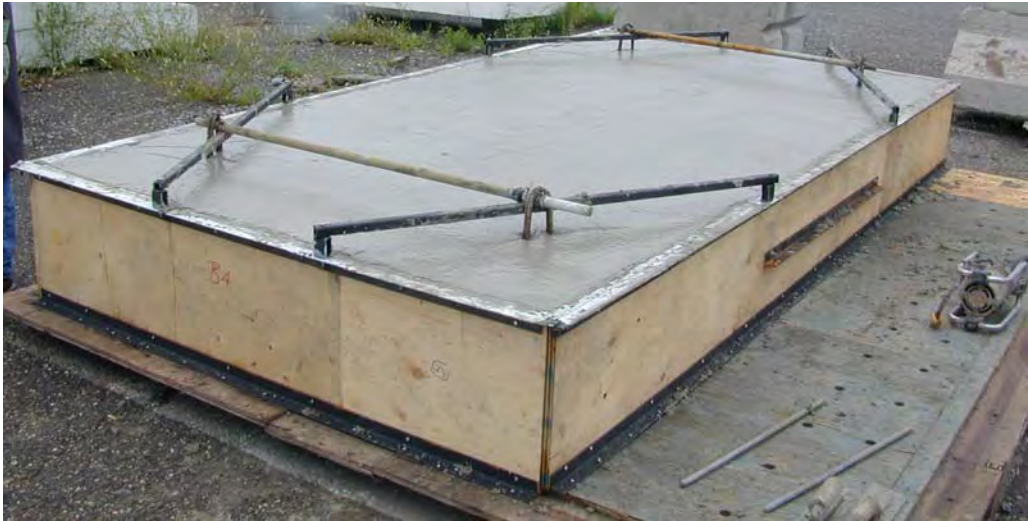
Figure 1: Concrete Slab after Casting
